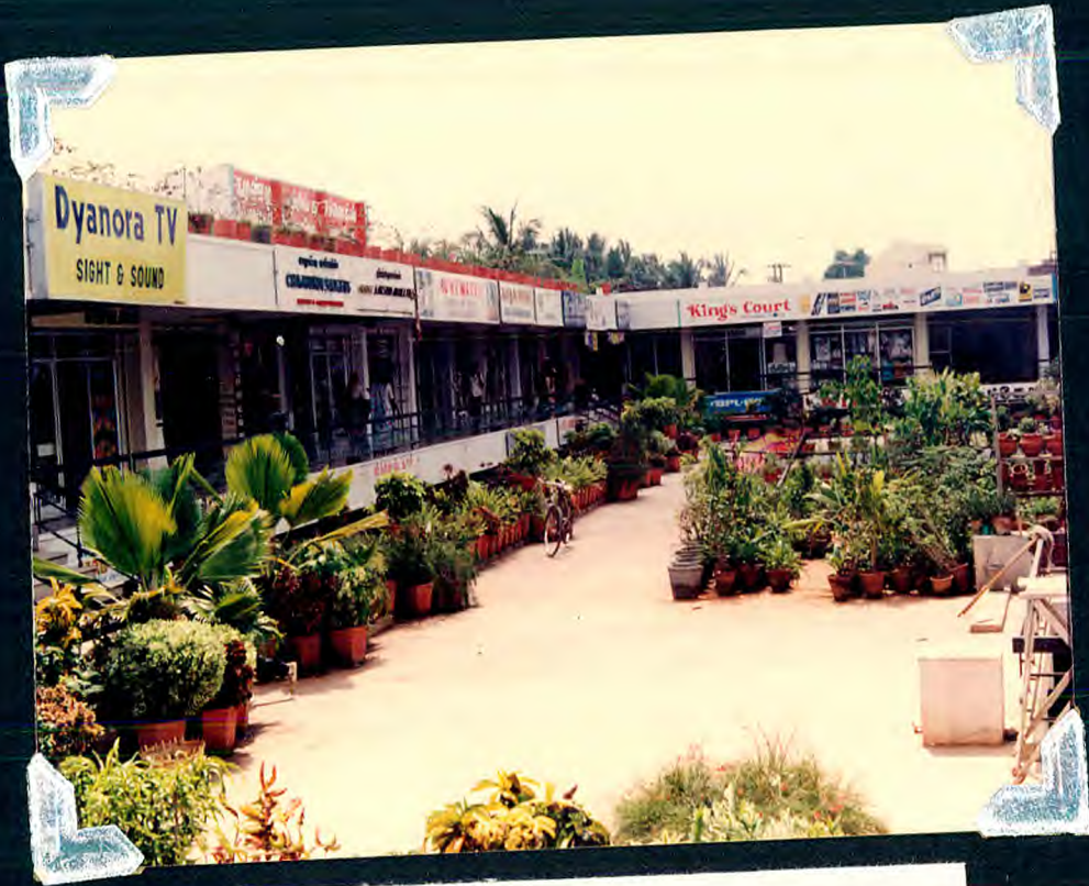
CHAMUNDI COMPLEX: FRONT VIEW
