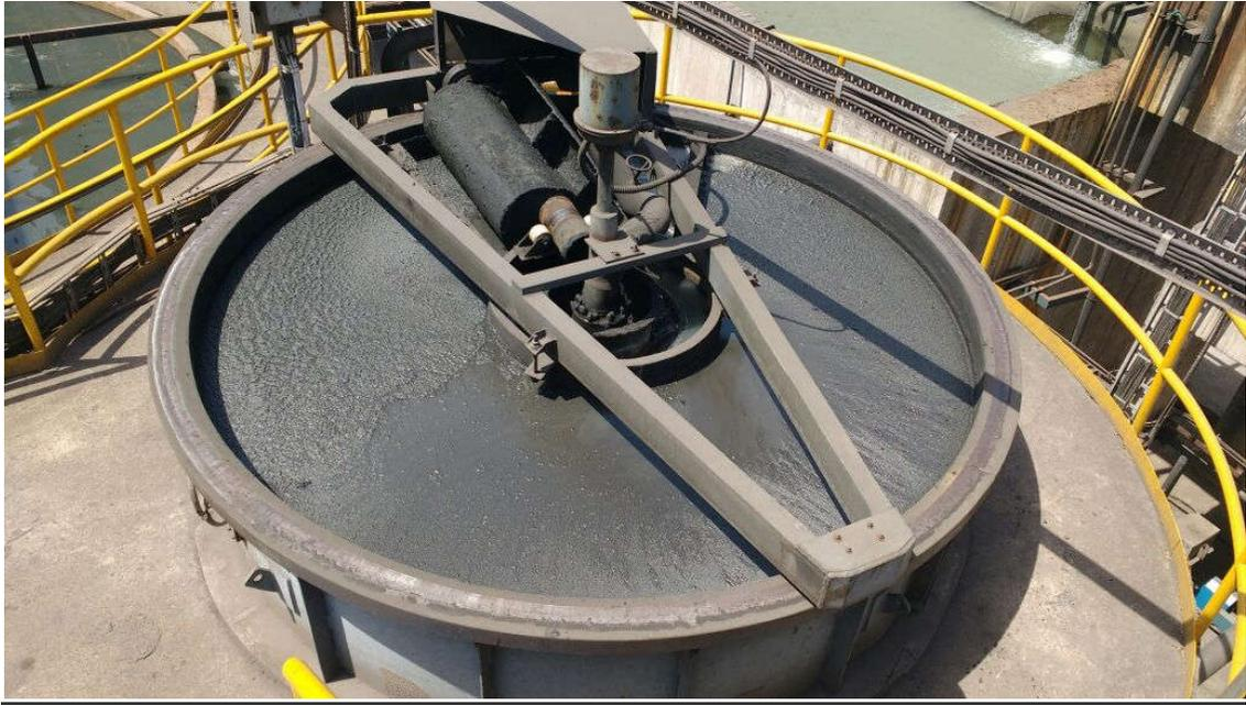
**Figure: 4.5 DAF System of WWTP at TATA Steel**
