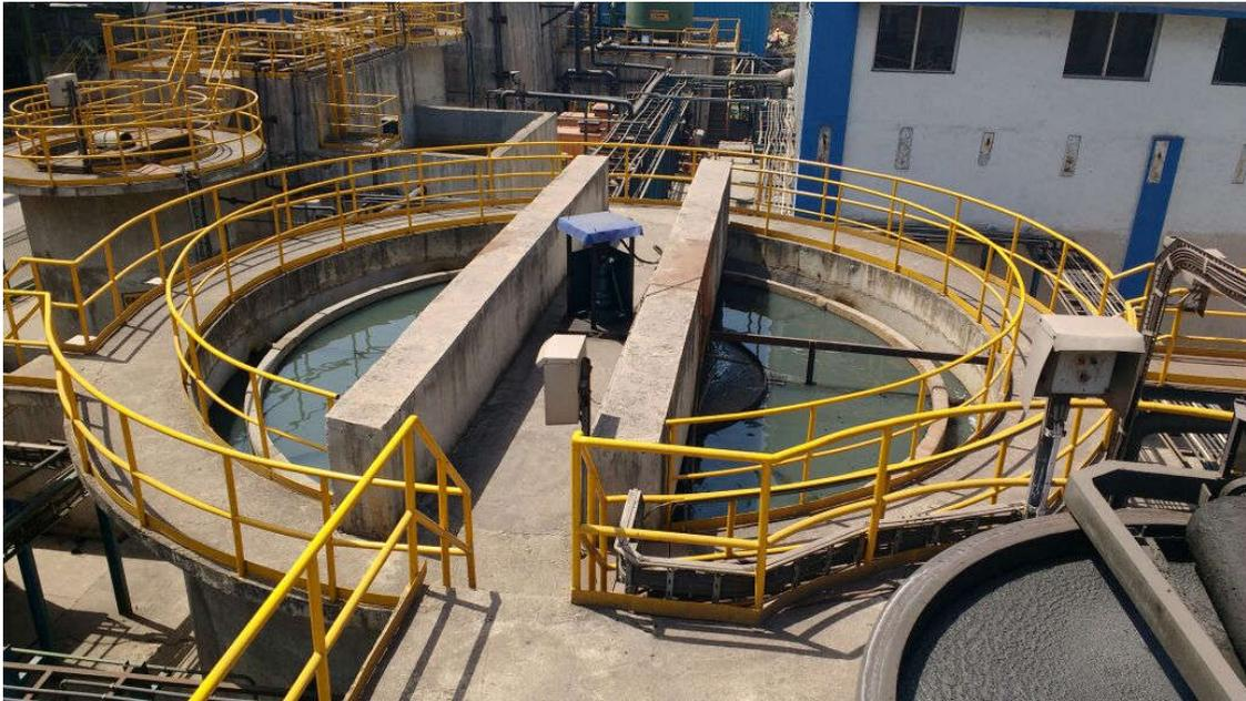
**Figure: 4.8 Clarifier Tank at TATA Steel,JSR; Blast Furnace WWTP Site.**
