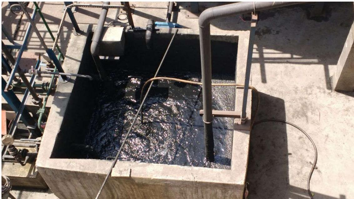
**Figure: 4.6 Effluent Water after DAF.**
