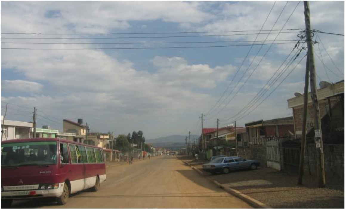
Plate-7.1 Collector Road without Foot Path
