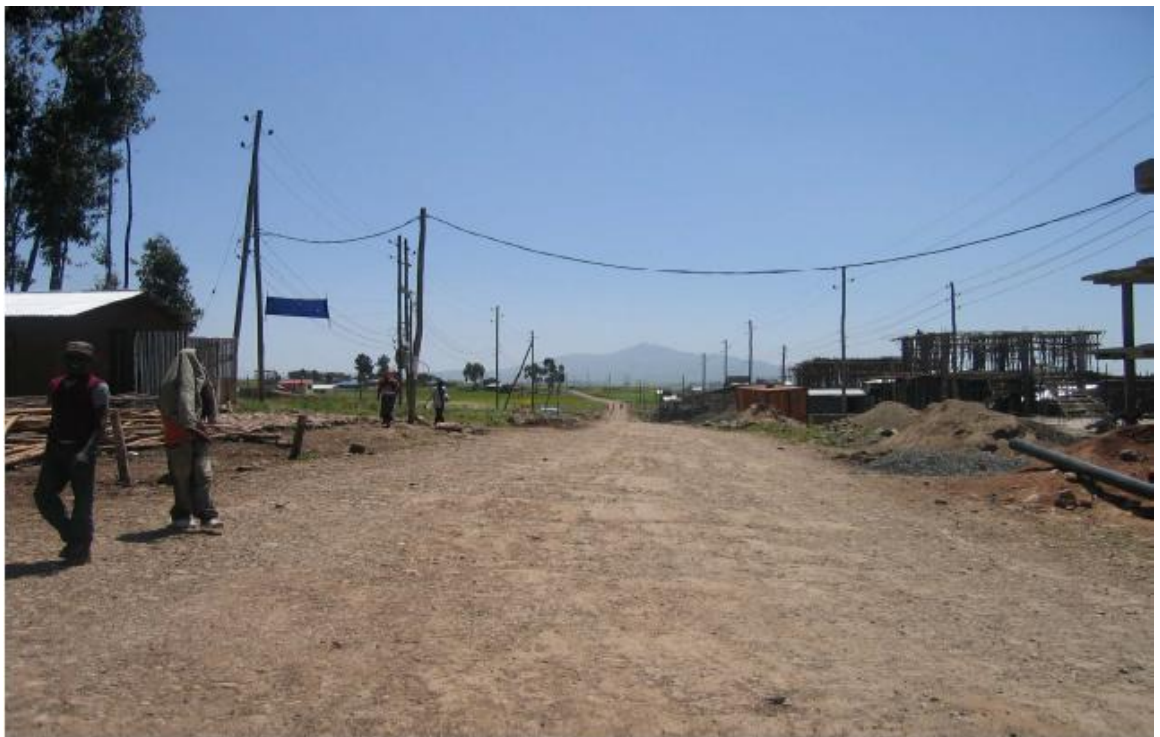
Plate-7.2 Gravel Road Provided with Neither Side Walk nor Drainage System (Peripheral Part of Yeka Sub City)
