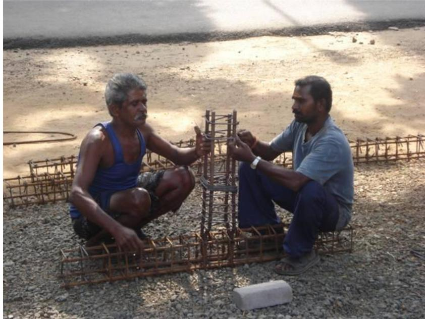
Fig.3.16 Typical View of Fabrication of Reinforcement
