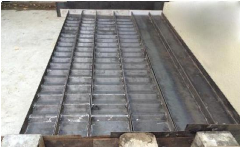
Figure 3.7 Specimens Before Concreting the Web
