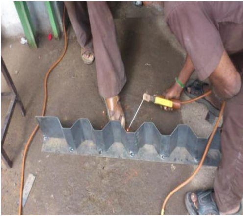
(c) Welding of the Corrugated Web with the Flange
